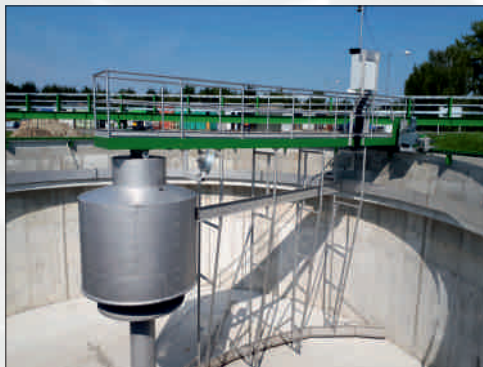
Vystrojení DN / equipment of secondary sedimentation tank
